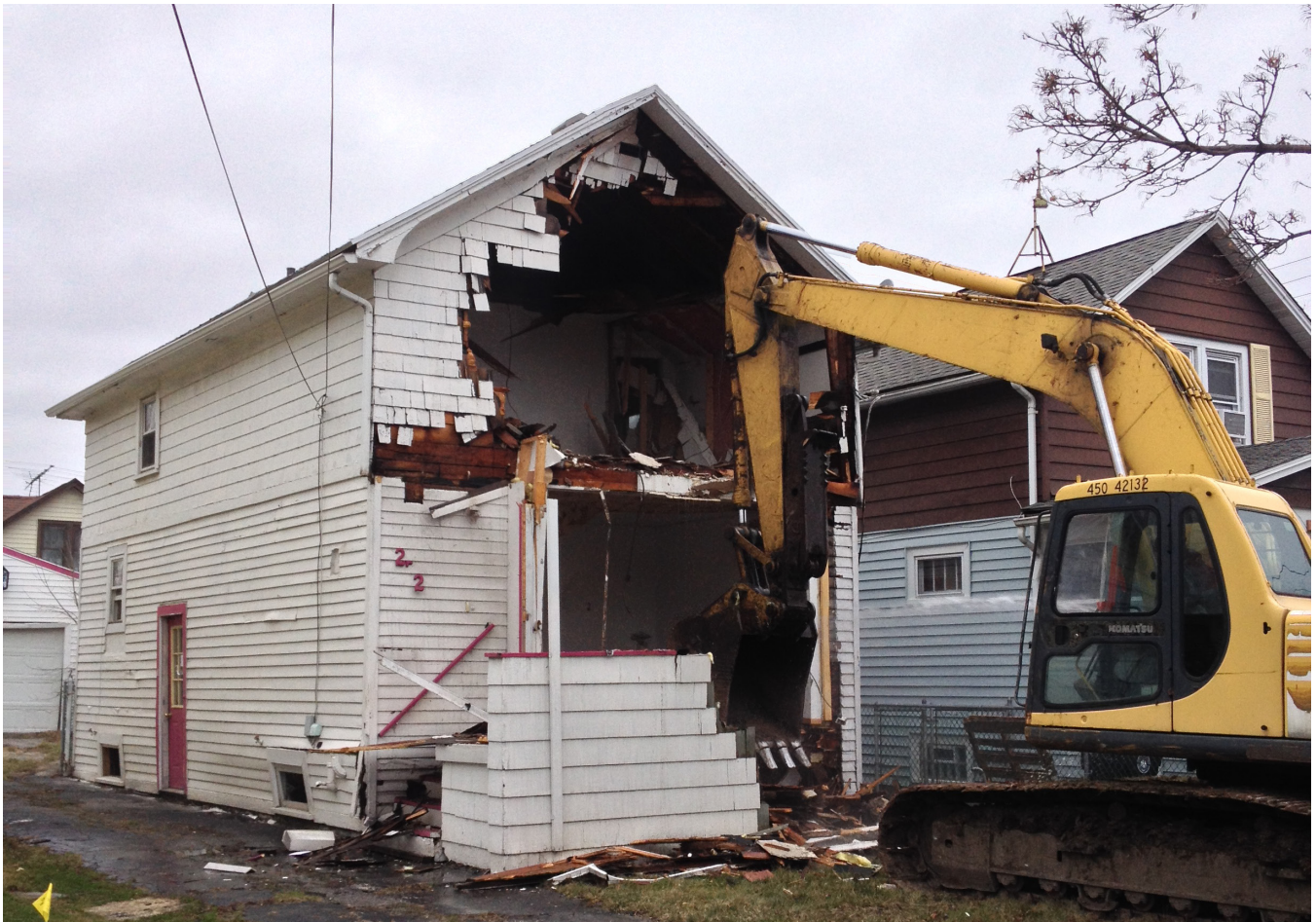
A demolition project in progress.
