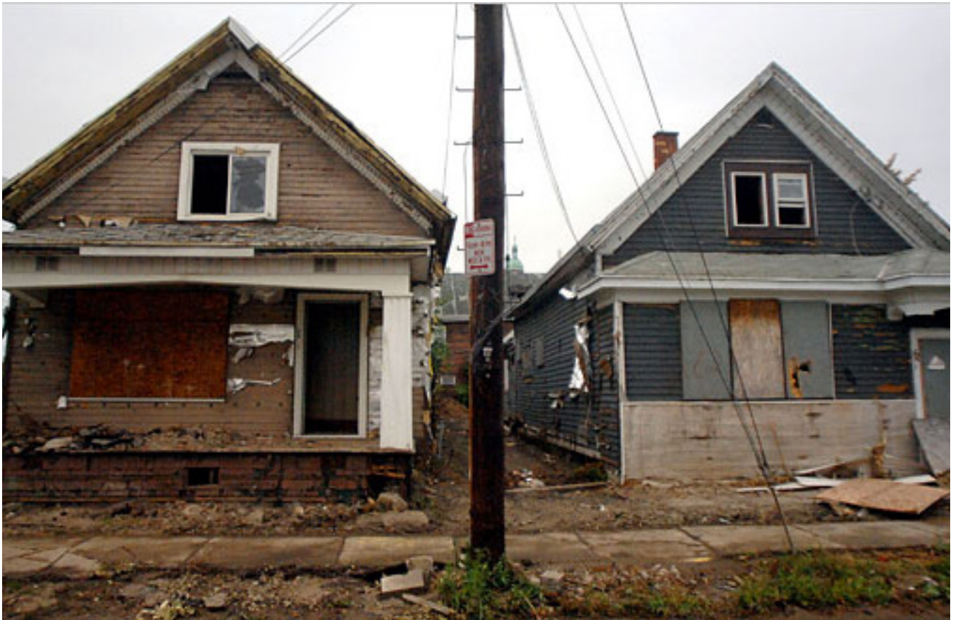
Vacant, dilapidated homes in BENLIC's service area.
