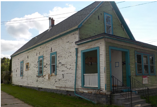
Before and after a BENLIC rehabilitation.
