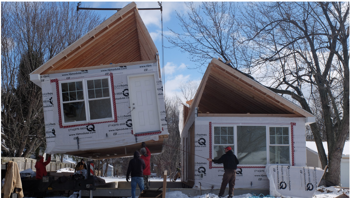
Modular construction infill housing.
