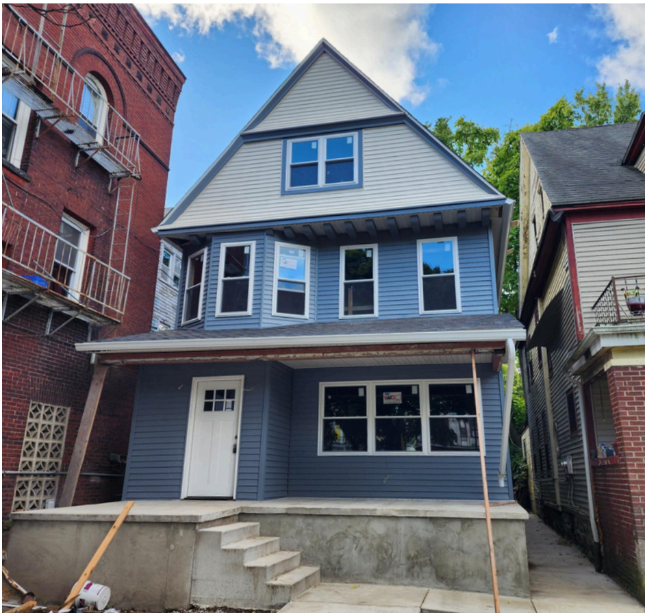
Progress as of 10/8/24
